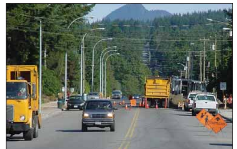
Paving work on Coast Meridian Road near Apel Drive.
